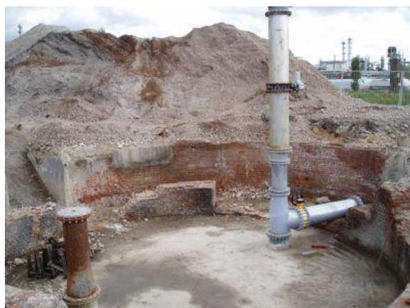
Fig. 1-5 : Example for a degassing pipe in a filled shaft
