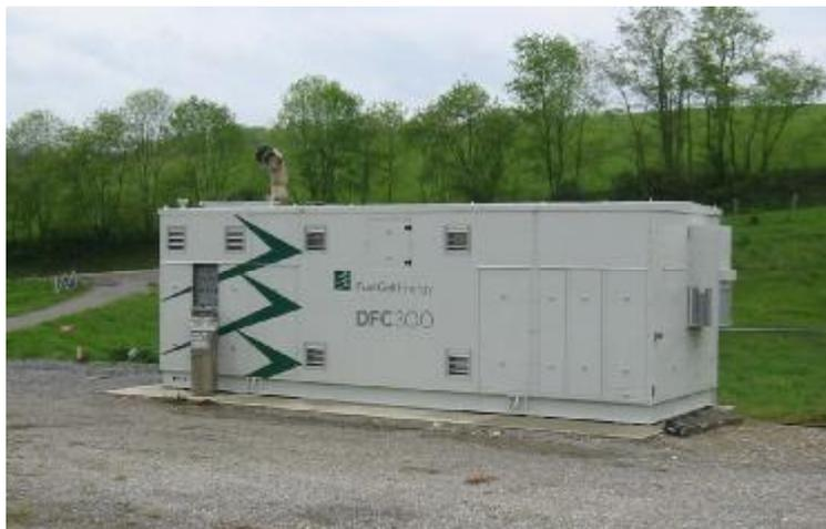
Fig. 8-2: 200 kW solid oxide fuel cell (SOFC) sited at AEP Ohio Coal LLC's Rose Valley Mine Site in Hopedale, Ohio. (Photo courtesy of FuelCell Energy Inc.)
