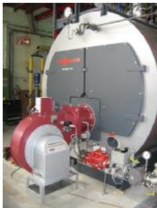
Fig. 3-2 : CMM burner with subsystems,
